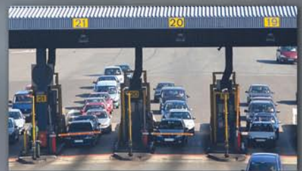
HIGHWAY SPEED TOLL COLLECTION
